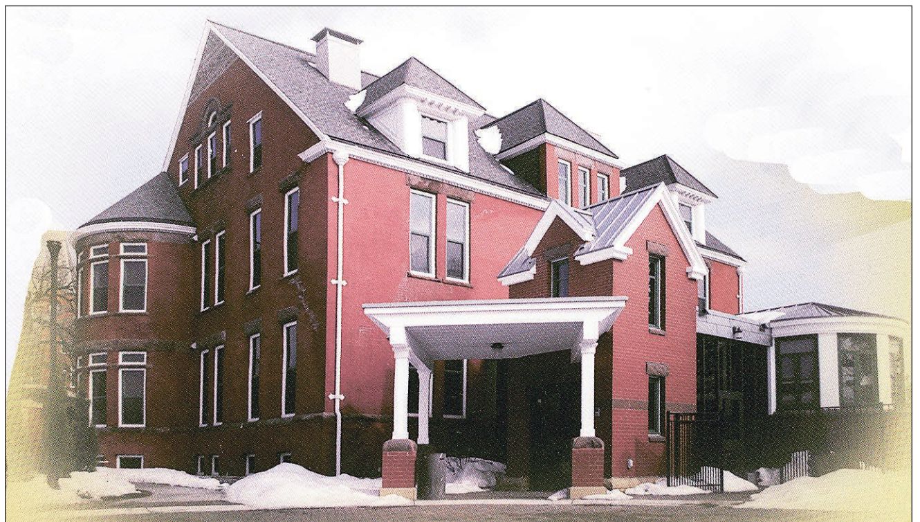
Building 4 is the oldest building on the Minnesota Veterans Home at Minneapolis, and it is housing the home's newest service, adult day care. The building was constructed in 1888 as a "cottage" for Civil War veterans. It has undergone an extensive $2 million remodeling which preserved the building's historic architecture and design while making it a comfortable, modern space for the center.
